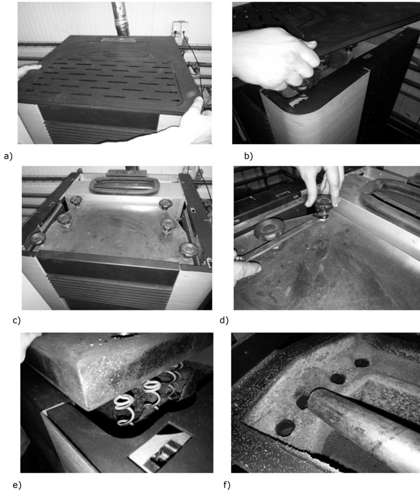
**Figure 43 - Cleaning the air flow pipes and turbulators**
