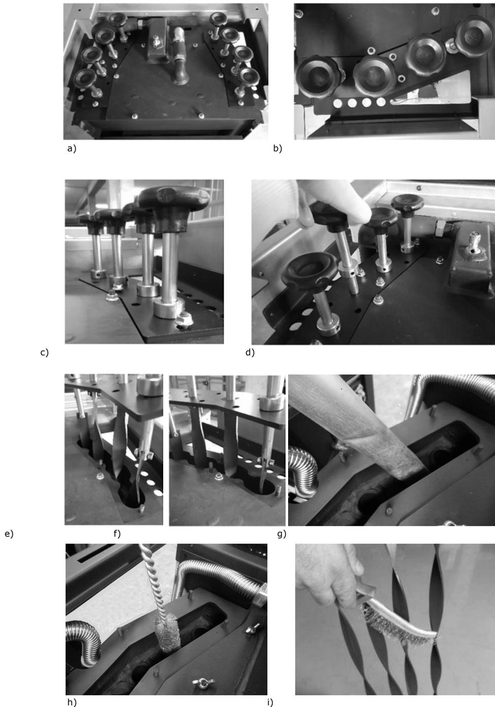
**Figure 44 - Cleaning the air flow pipes and turbulators**
