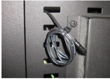
Figure 14 - Room temperature probe
